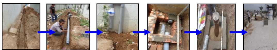
Figure. 5: Digging of ground
