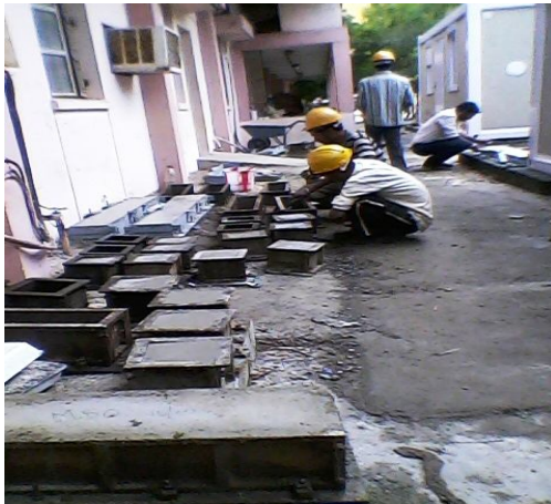
Figure: 1 Casting of Specimens
